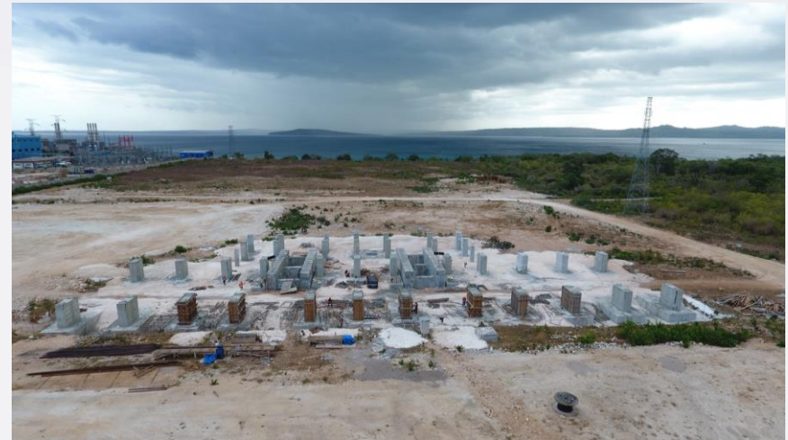
Figure 3: Concrete Foundations Finished at Smelting Hub Facility
